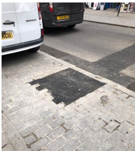
Setts replaced by tarmac concrete blocks
