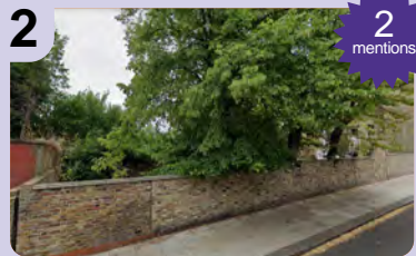
2 Gap between building identified as a small site that could improve antisocial behaviour. This site received an agreement.
