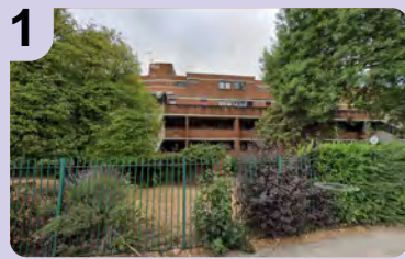
1 While this would not be classified as a small site Charlton Court was identified as having potential to be redeveloped as more housing.
