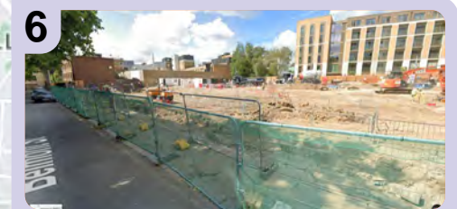
6 Building site of forthcoming Charlie Ratchford Court.
