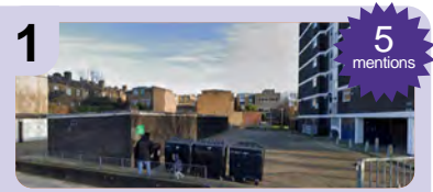
1 The garages in front of Monmouth House were identified as a potential site that could be more well used and see a reduction in anti social behaviour. This site forms part of the Local Conversations on Raglan Street Estate
