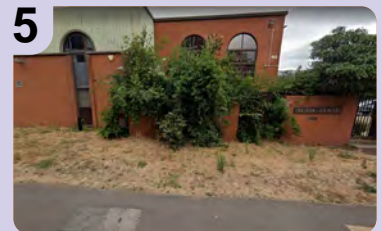
5 Alpha house and surrounding area identified as having potential to be more well used. This site received an agreement.
