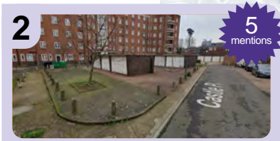
2 Castle Road Estate is a Local Conversation site. The garages in the centre of the estate were identified as a potential site that could be made more attractive through a small sites build.
