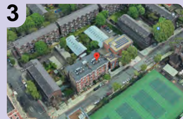
3 A hardstanding area near Kingston House on Camden Street was identified as an area that could be more attractive and better maintained through a small housing project.
