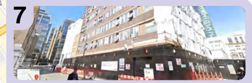
7 While this building would not be classified as a small site it was identified as a space that could be more attractive, more family/child friendly and better maintained if it was used as a small site.
