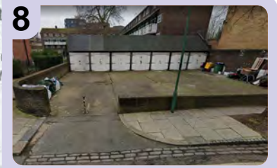
8 Lock up sheds beside Victory House on Clarence Way identified to allow for a better use of space. This site received 2 agreements.
