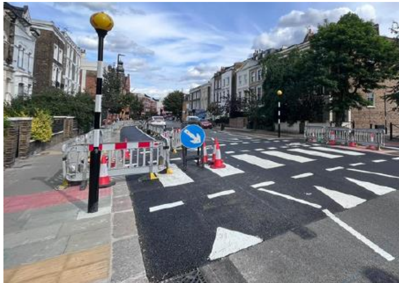
Image 38: Prince of Wales Road nearly complete
