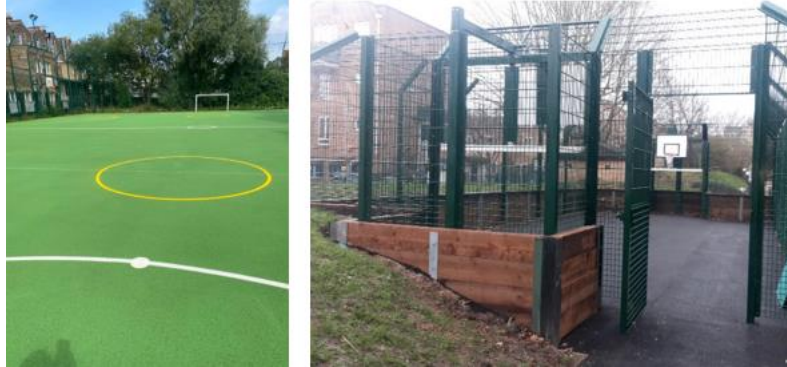
Images 11&12-Refurbished Ball courts: Kilburn Grange and Jim's Pitch (Russell Nurseries)
