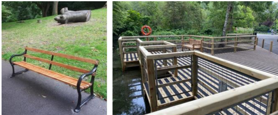
Image 13&14- Restored benches using local timber and restored pond decking (Waterlow Park)
