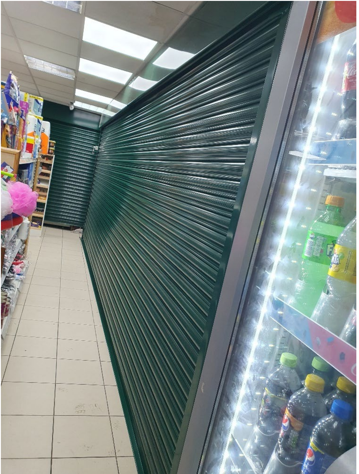
(4) Photographs of shutters in place
