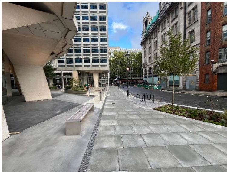
Kemble Street pavement improvements and urban
