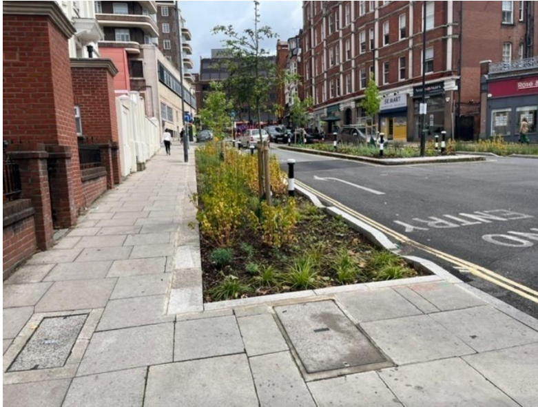
Figure 3: 2024 SuDS scheme in Goldhurst Terrace (image)
