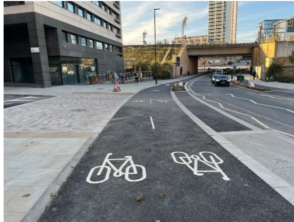
York Way permanent scheme under construction (Autumn '24)
