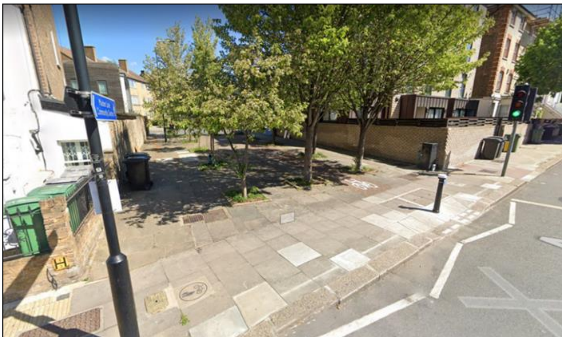
Figure 2: A dropped kerb and removal of pedestrian guard railing provides improved access for cyclists and improves the street scene
