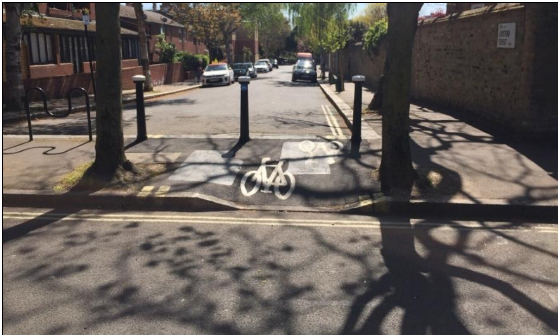
Figure 1: A dropped kerb and ramp on the pavement allows cyclists to travel more easily between Linstead Street and Netherwood Street
